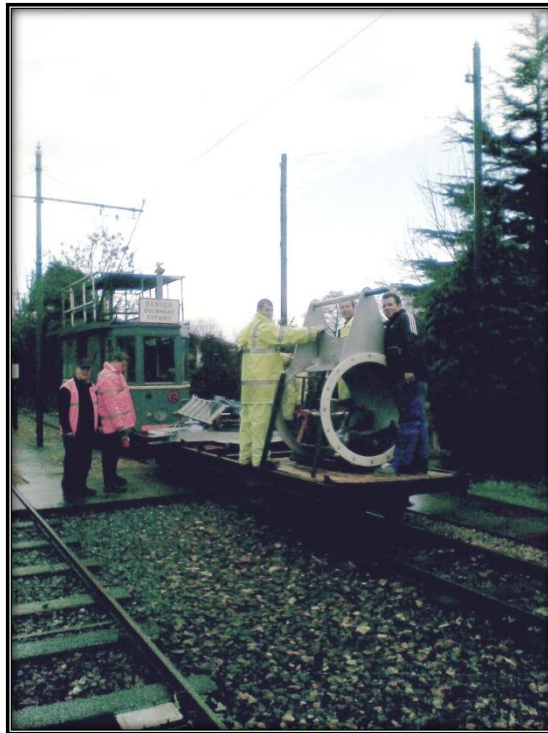
The above image shows the valve being loaded onto the tram for transportation to site location.
